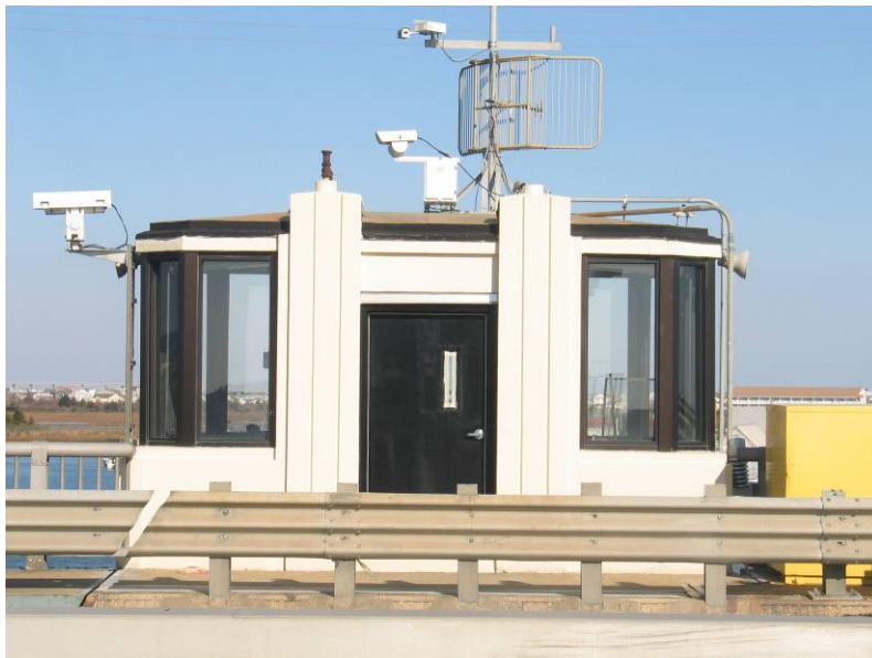
Figure 1 - View of North Tower
