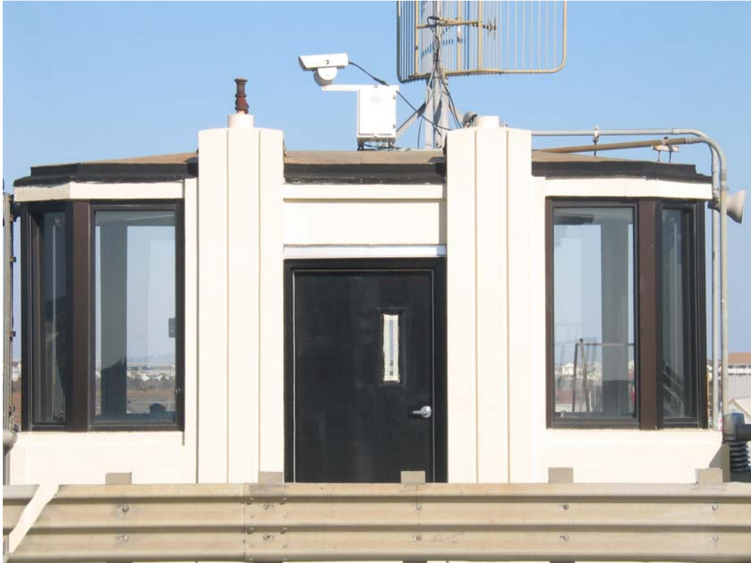
Figure 2 - View of North Tower – Close-Up
