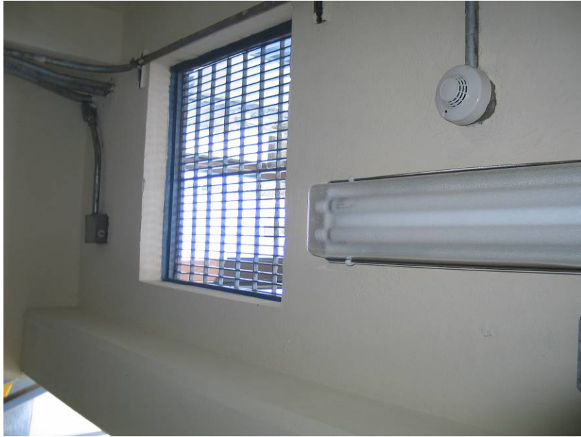
Figure 4 - Details Near Fixtures (North Tower)
