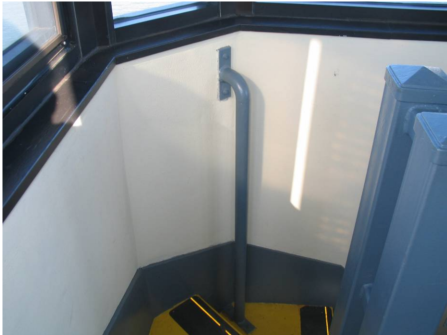
Figure 5 - Details Near Steps (South Tower)
