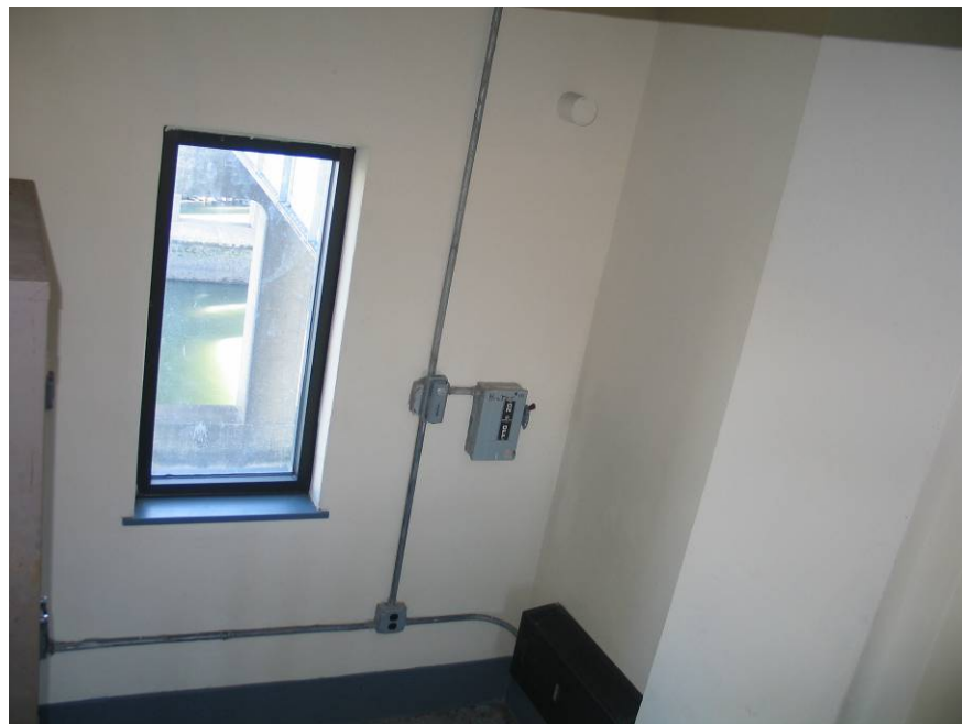
Figure 3 - Finished Inside Surface Including Treatment Around Window (North Tower)
