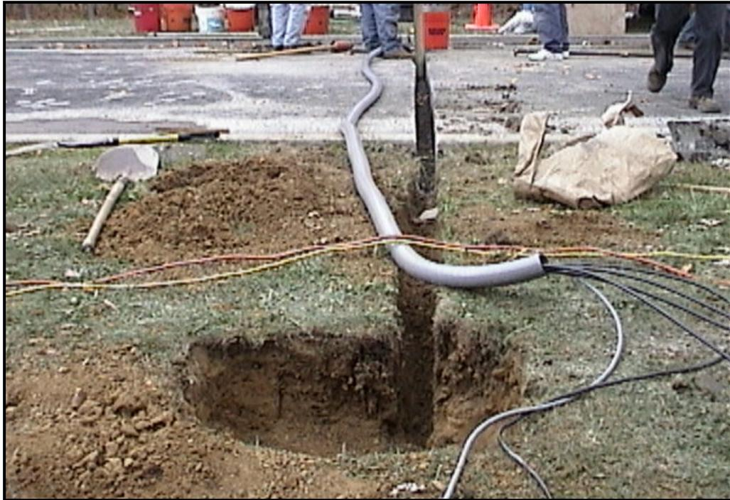
**Figure E.5: View of Trench with Equipment Cabinet Hole in Foreground**
