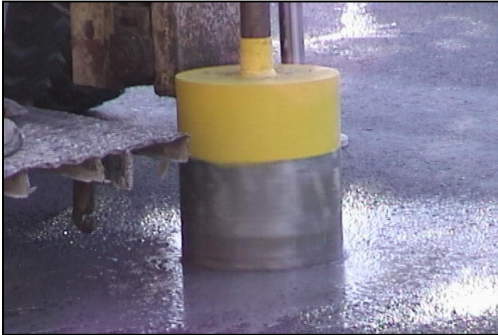
**Figure E.1: Coring the Instrumentation Hole**
