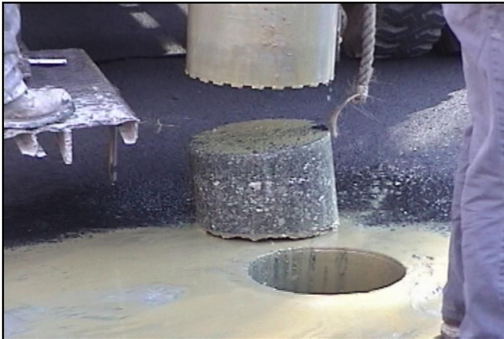
**Figure E.2: Removing the Instrumentation Hole Core**
