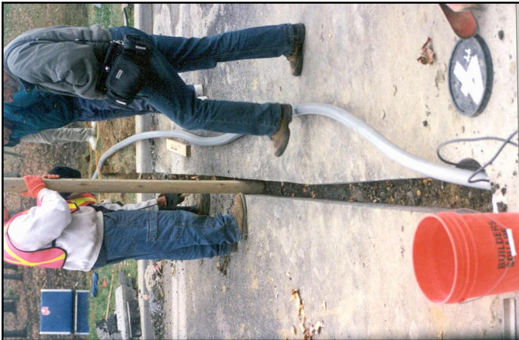
**Figure E.6: Compacting the Trench before Laying the Conduit**
