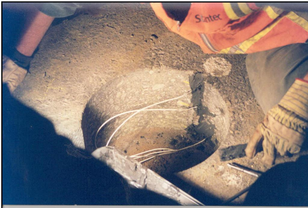
**Figure E.4: Installed MRC Pavement Probes**
