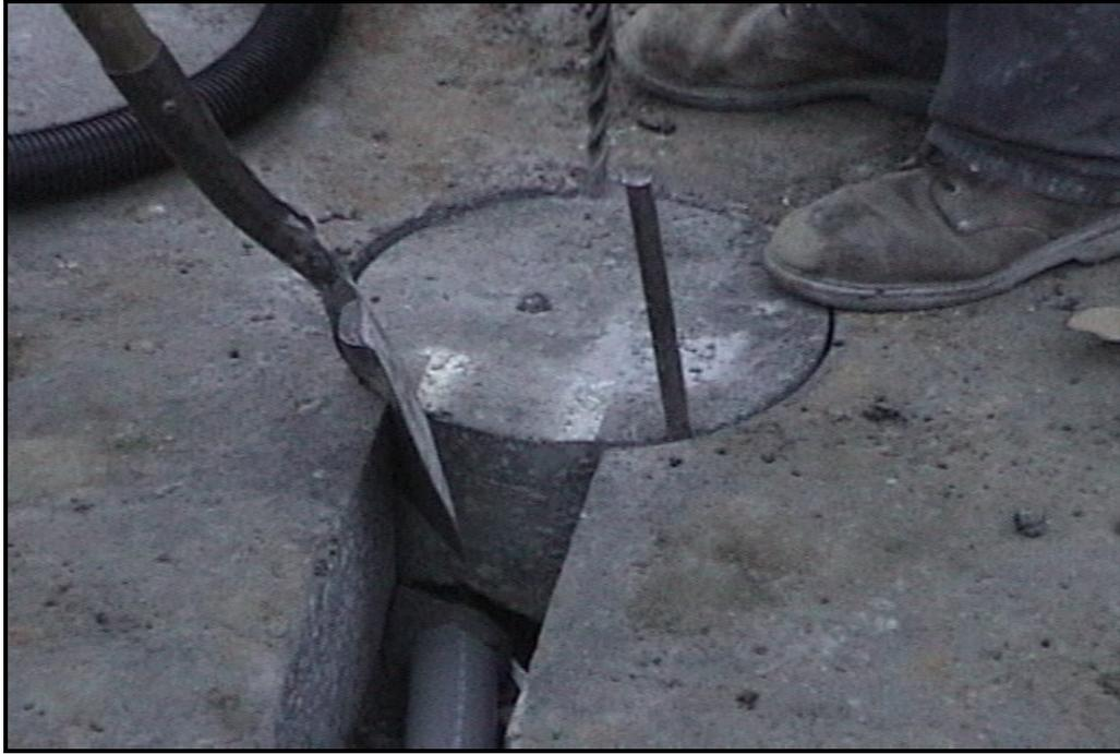
**Figure E.7: Replacing the Instrumentation Hole Core**
