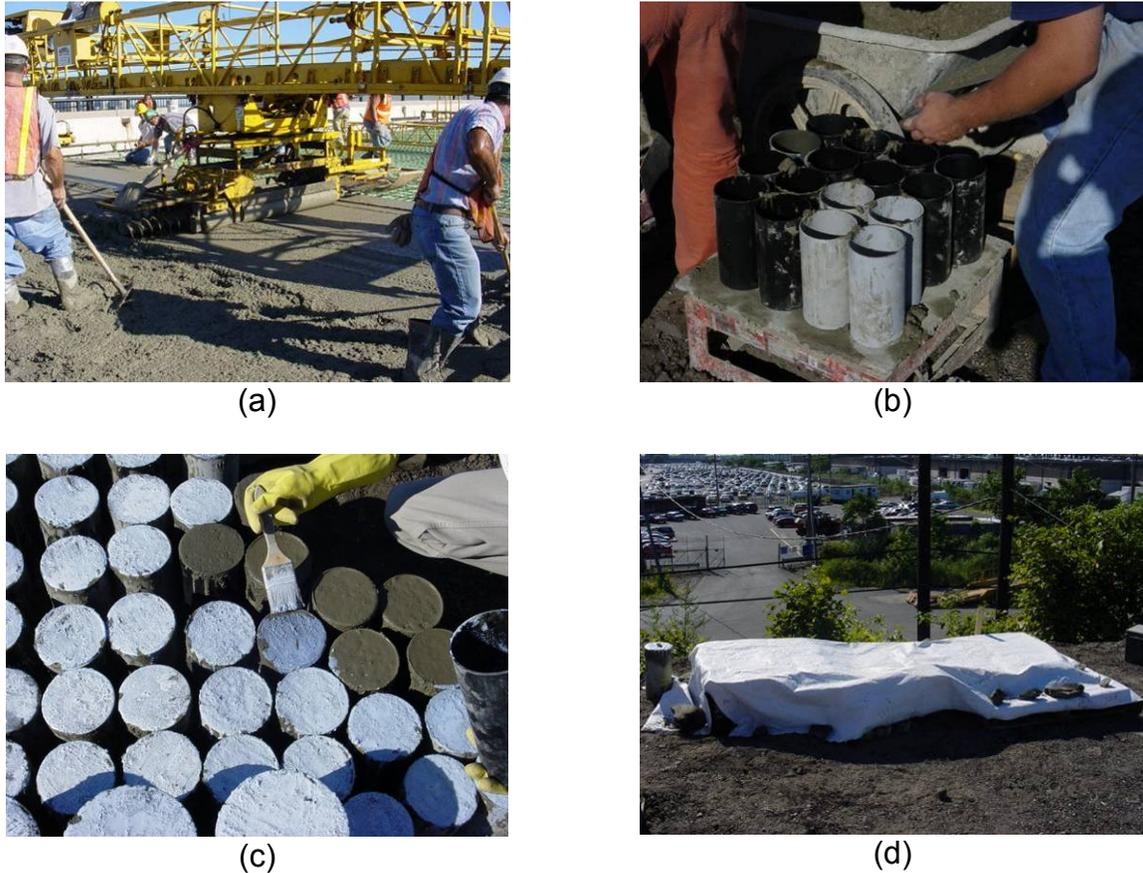
Figure 13. Concrete sampling: (a) pouring deck slab, (b) consolidating specimens, (c) applying curing compound, and (d) covering specimens with wet burlap
