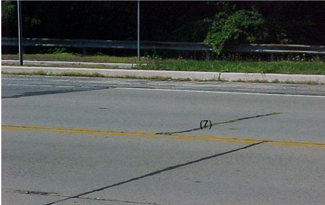
Figure 64. Photograph of a transverse crack in right lane, at exit on bridge # 14.
