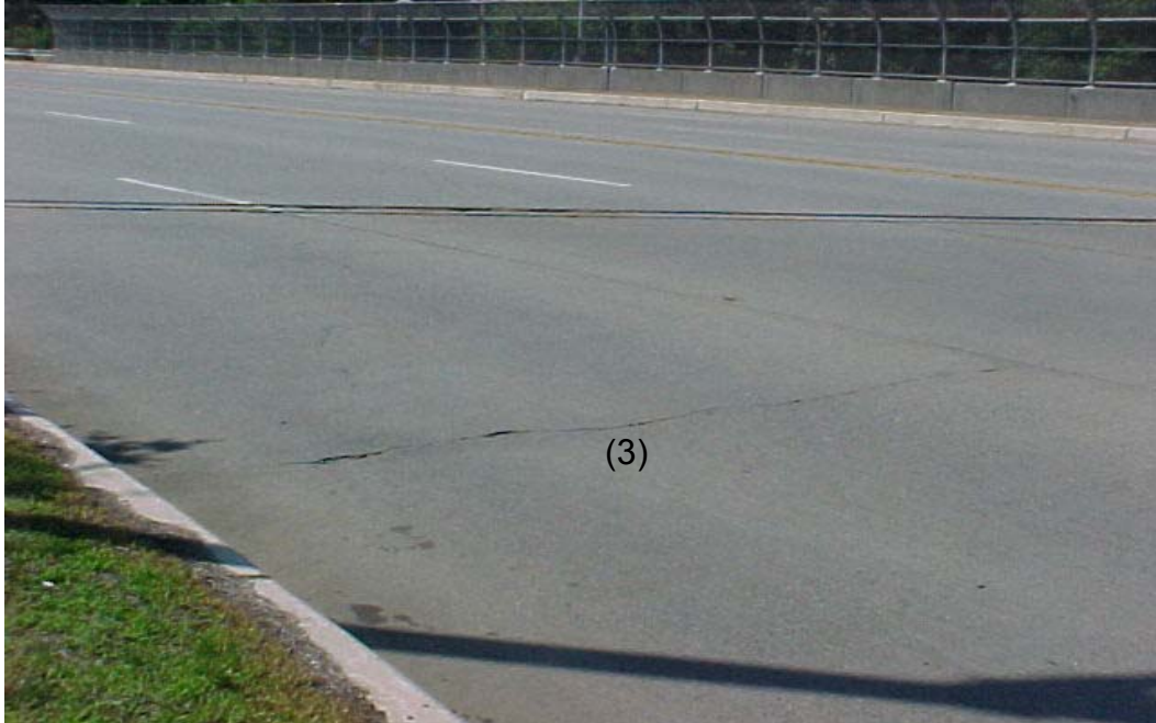
Figure 60. Photograph of a transverse crack in right lane, at exit on bridge 14.
