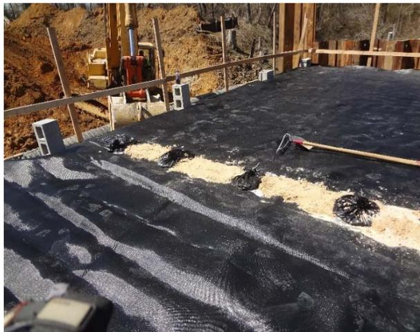
**Figure 3.10 Strain gauge protection and installation at the site**
