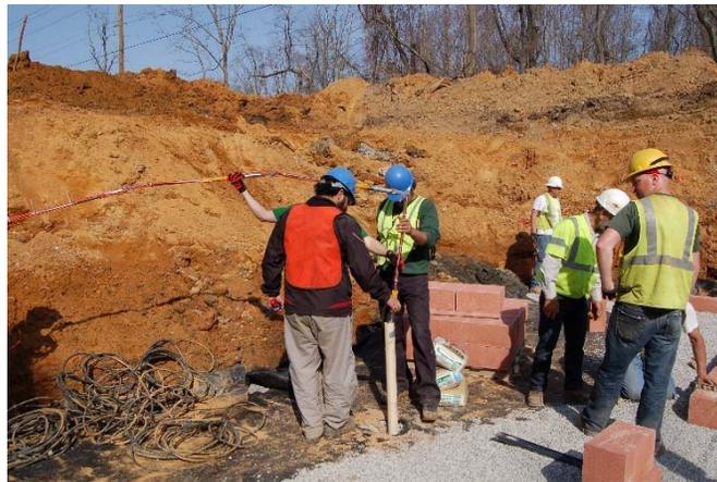
**Figure 3.3 IPI sensor array installation**
