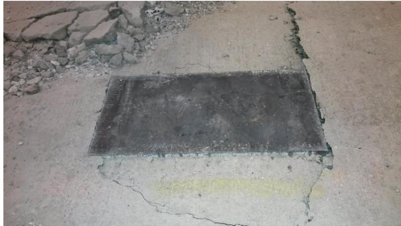
Figure 3.36 Tire contact area plate embedded in deck
