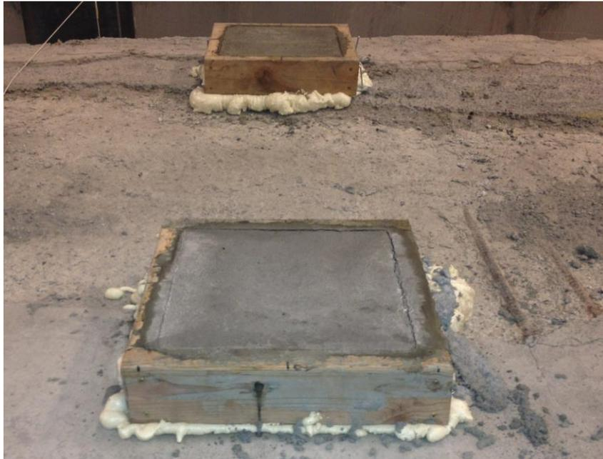
Figure 3.14 Typical concrete leveling pads
