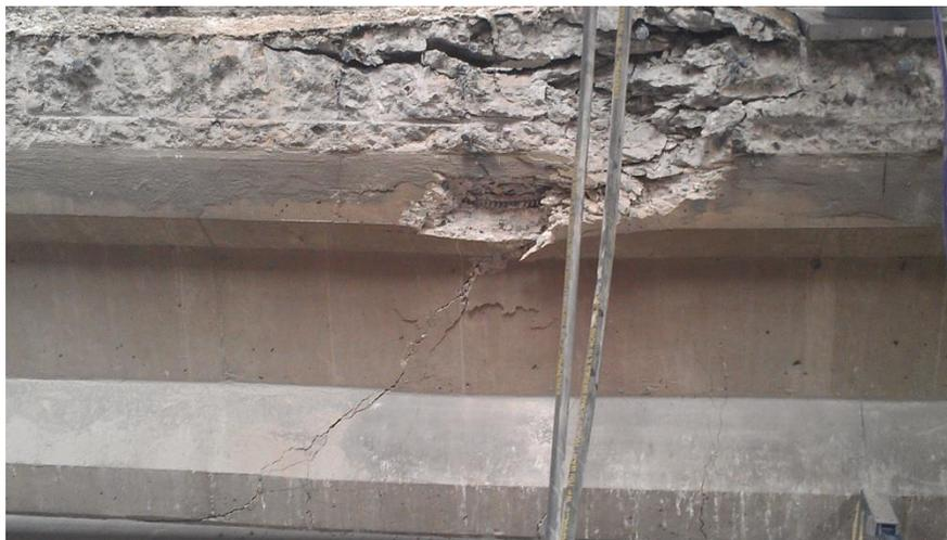
Figure 29 Shear failure in G1-2d(a)
