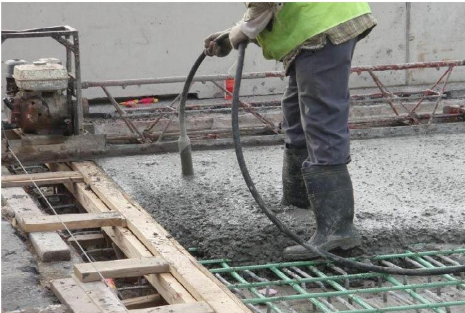
Figure 2 Internal Concrete Vibration (Image Source - Wikipedia.org)
