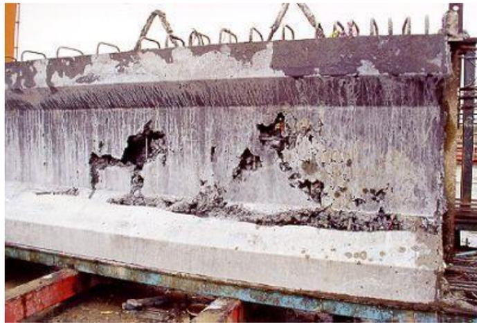
**Figure 1 Honeycomb defects in concrete caused by improper consolidation**
