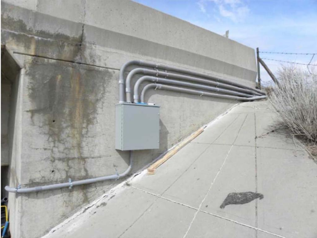
*Figure 4.2 Junction box located on abutment wing-wall*
