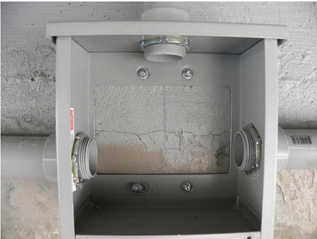
*Figure 4.3 Junction boxes showing water-tight fittings*
