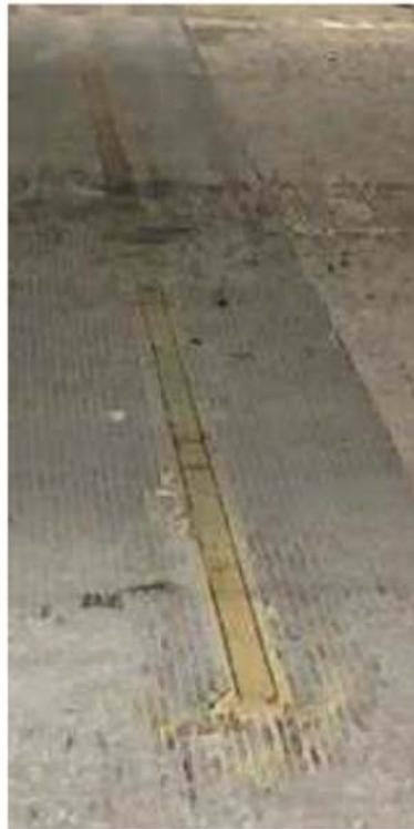
*Figure 3.2 Quartz based WIM installed in lane leading to Perry Utah Port of Entry*
