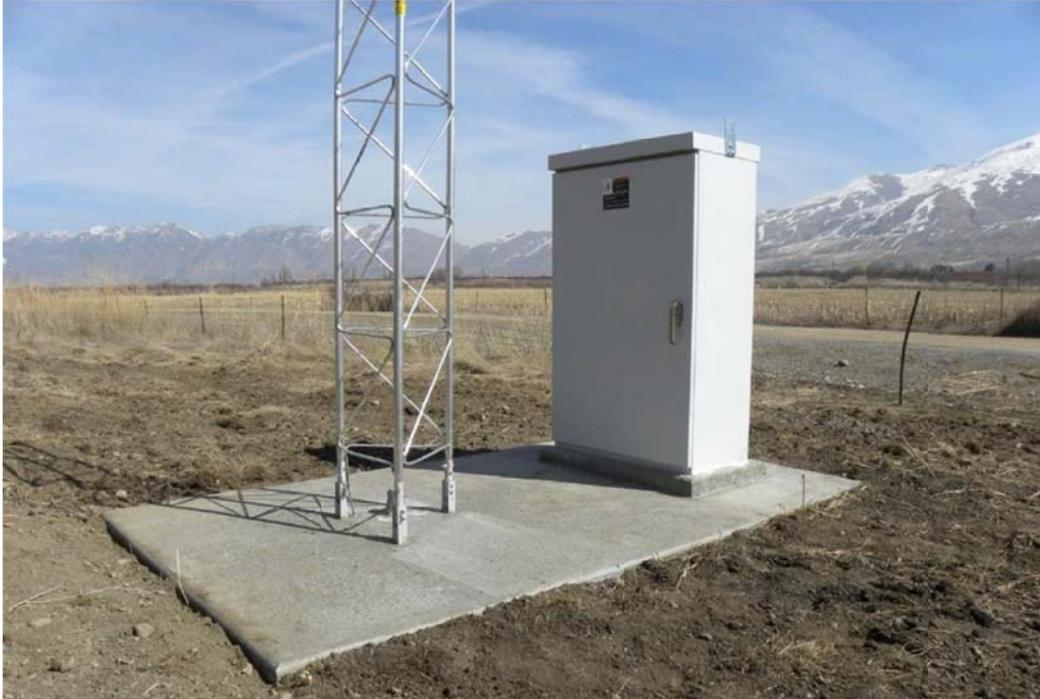
*Figure 4.1 Instrument pad with installed tower and cabinet after grading*
